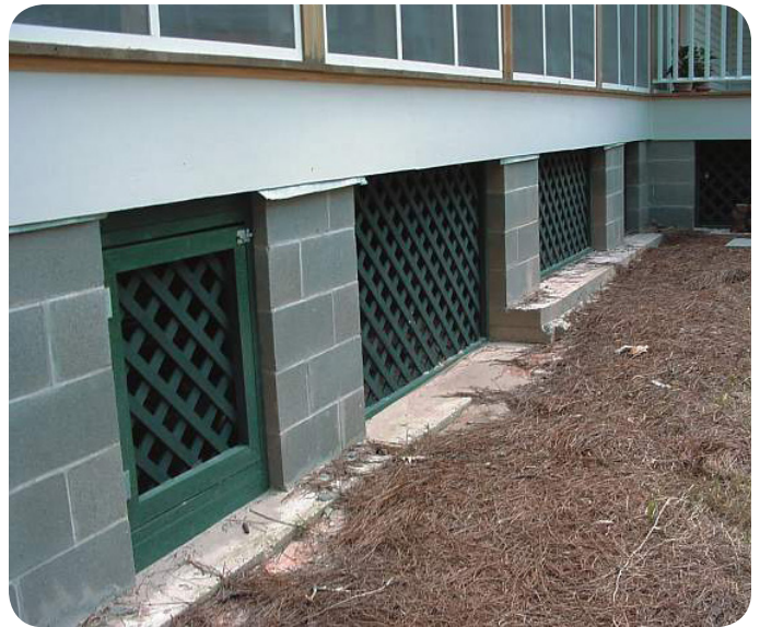
Figure 3.2: Crawlspaces allow floodwaters to flow through the building
