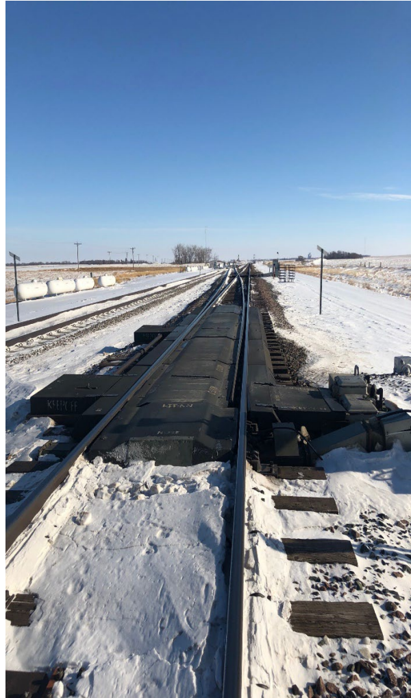
Fiberglass Switch Heater Covers
