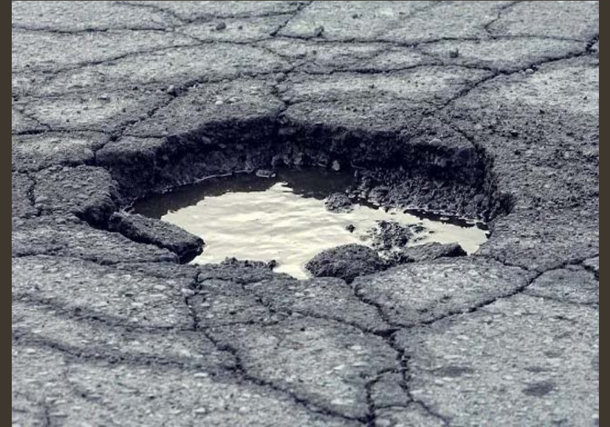
Load Failure
