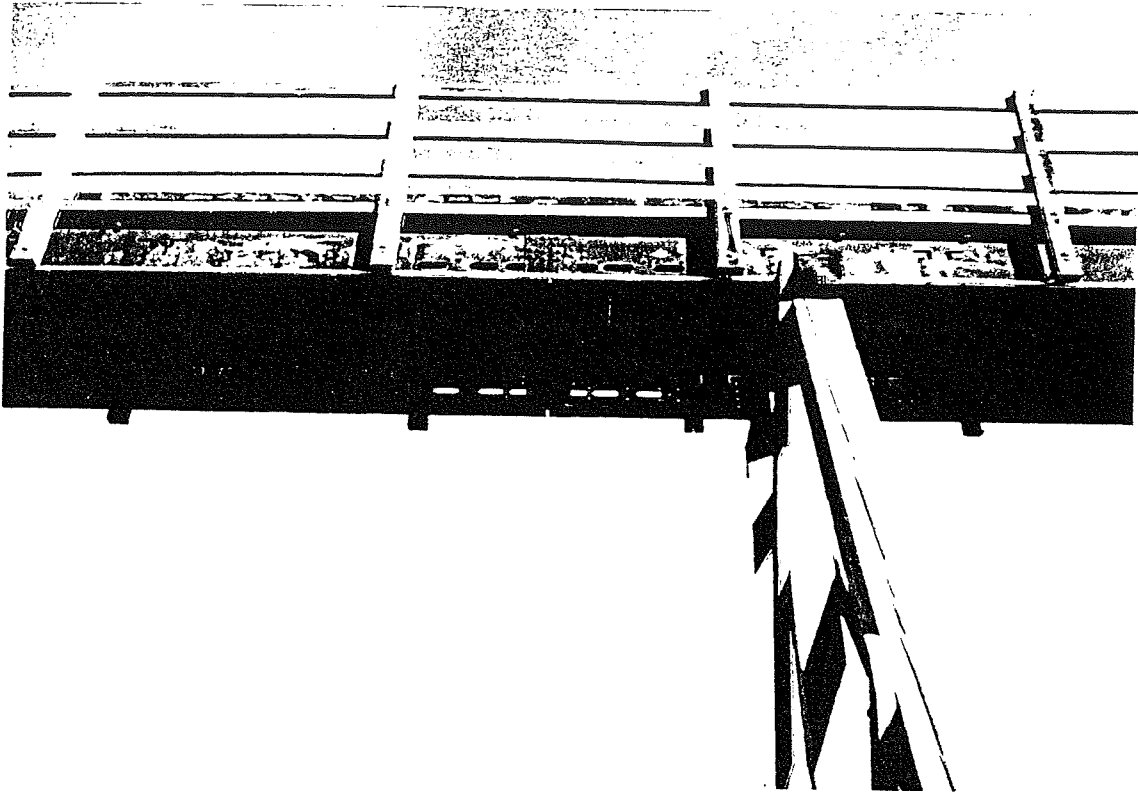
BR. 202.8 STAMP ON STEEL GIRDERS NEAR B16 (TYPICAL AT EITHER SIDE OF TRUSS)
