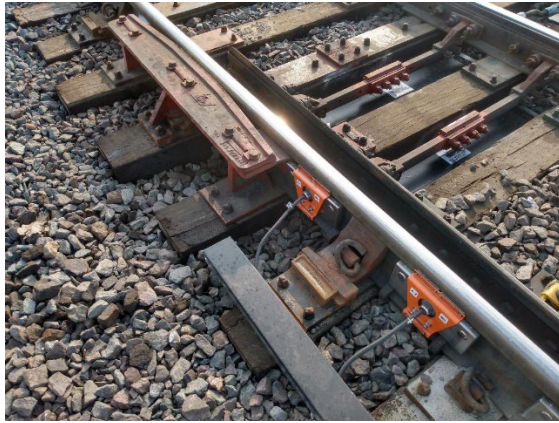
Installation photos of Hot Switch Heating Systems on the Rail
