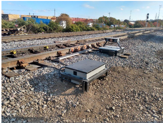
Installation photos of Hot Switch Heating Systems on the Rail
