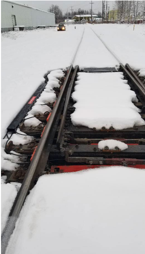
Hot Switch Heating System
