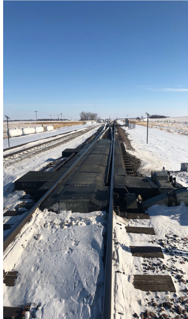
Fiberglass Switch Heater Covers
