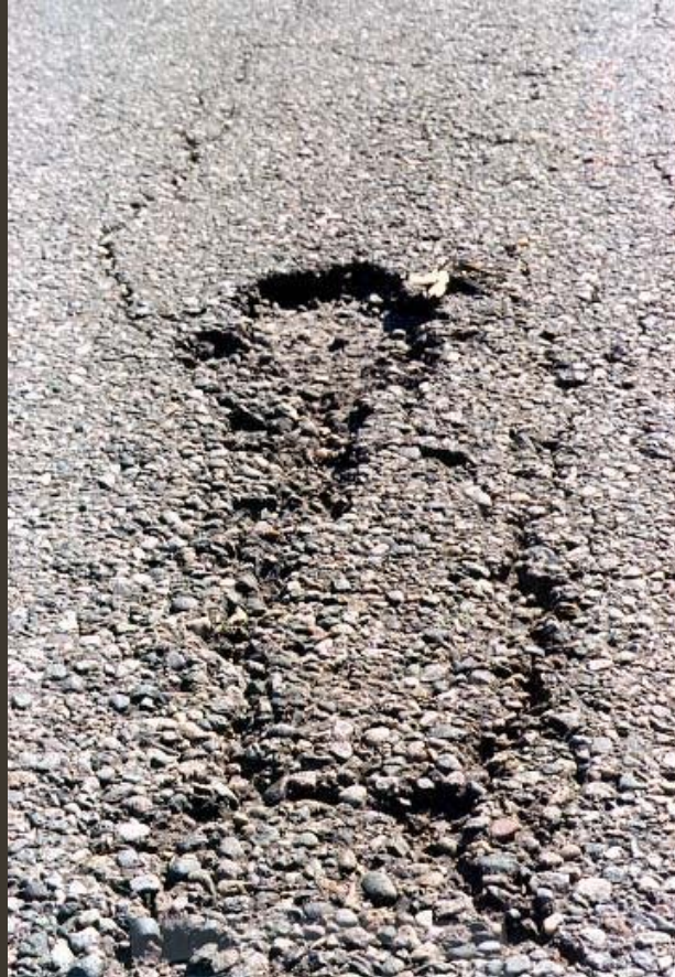
Weathering Failure
