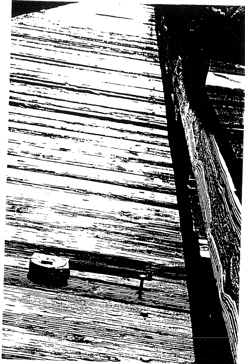
BR. 202.8 LOOSE NAILS IN TIMBER DECK PLANK (TYPICAL)
