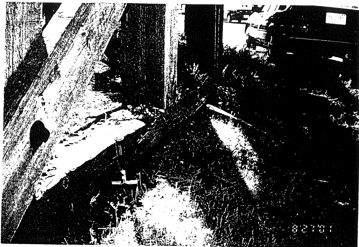
BR. 202.8 DECAYED & CRUSHED FOOTING TIMBER ON B12
